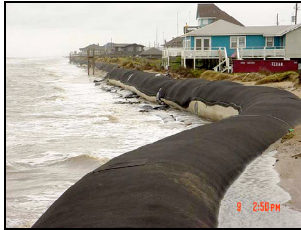
Sandsock, sand-filled tubular geotextile (Source: Surfrider Foundation, 2006)
