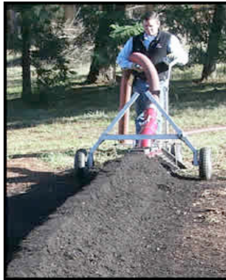
Installation of compost berm (Source: Rexius, 2006)
