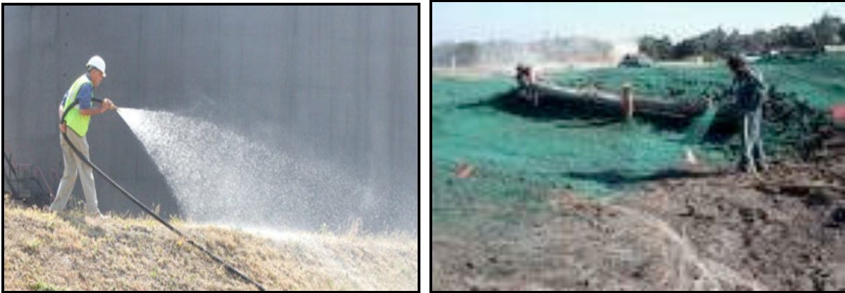
Hand application of hydroseed on construction sites (Source: RMB Craftscapes Ltd, 2006)
