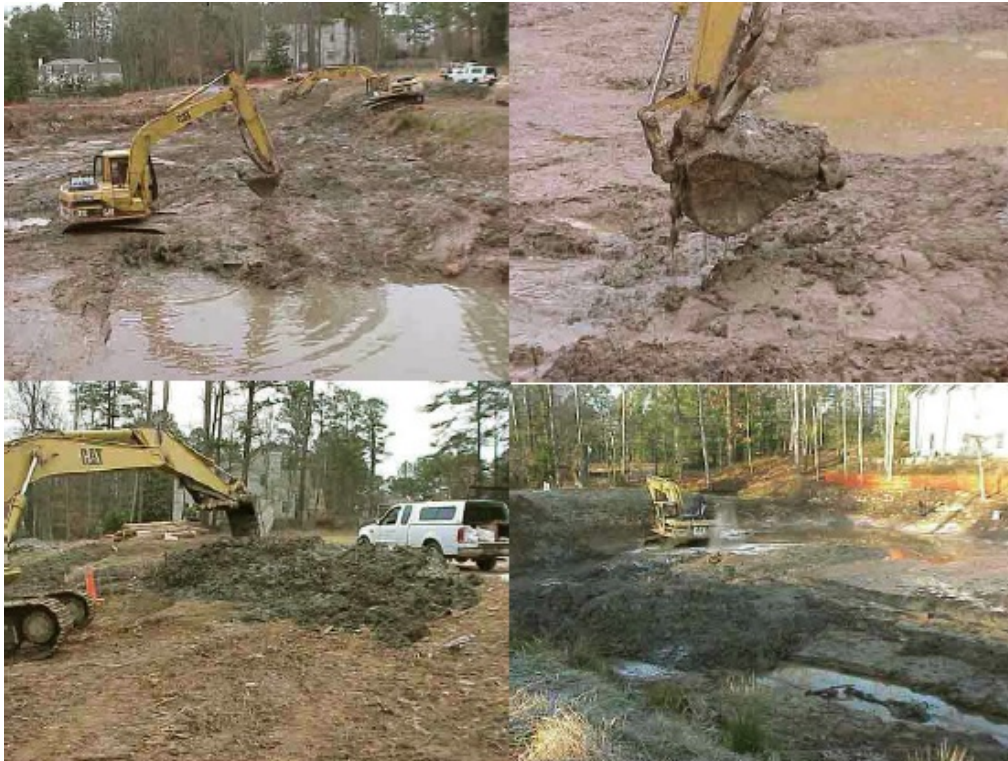
Figure AIII-28: Polymer-enhanced Mud and Sediment Removal.
