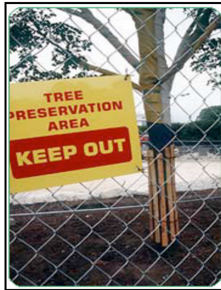
Marked tree preservation area in construction zone (Source: National Gallery, 2006)
