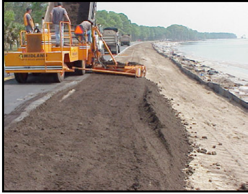
Placement of compost mulch layer
