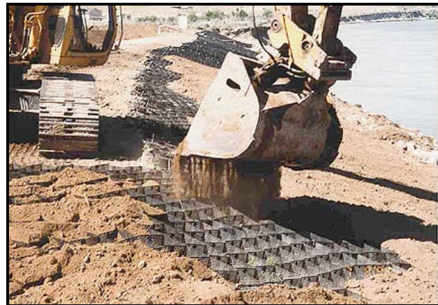
Metal geogrid being installed for beach stabilization (Source: IECA, 2006)
