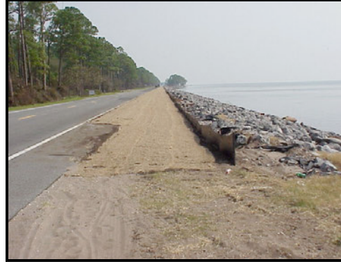
Placement of jute fiber erosion control blanket
