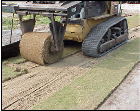
Placement of bermuda grass sod over jute blanket
