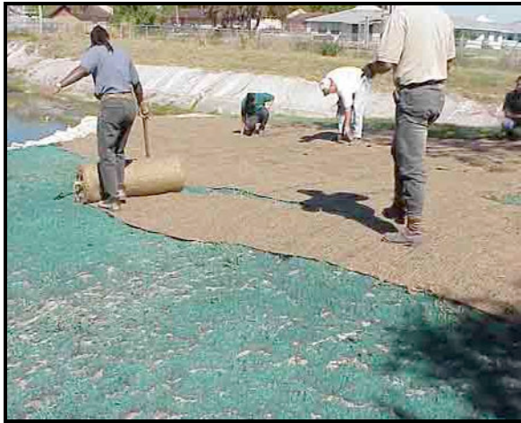
Jute fiber geomat in Broward County, FL (Source: Applied Polymer Systems, 2000)
