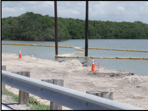
Turbidity barrier along US Hwy 1, Key Largo, FL (Source: Molly Wood, 2006)
