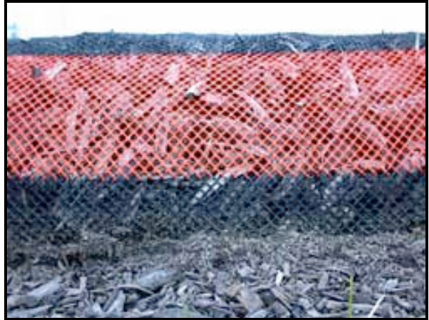
Detail of compost-filled mesh sock (Source: Filtrexx, 2006)
