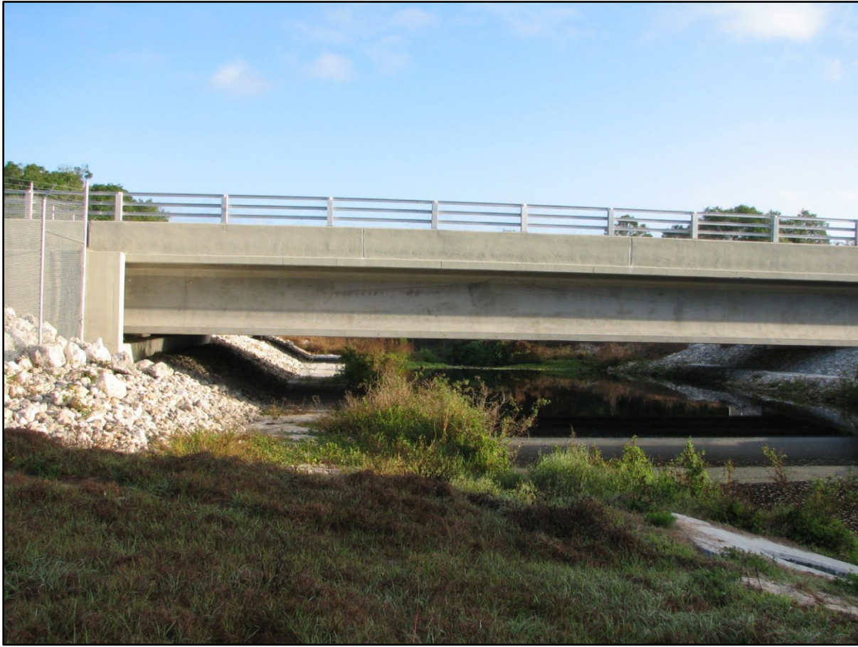
Figure 17 – 1 Bridge with Shelves for Wildlife
