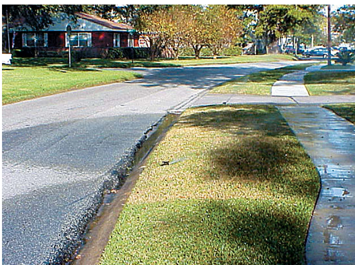
Figure 12. Poor design; sprinkler does not match area.
