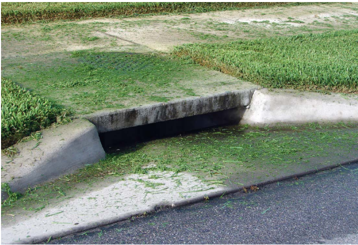
Figure 8. Always remove clippings from impervious surfaces. These nutrients are going straight to a water body.
