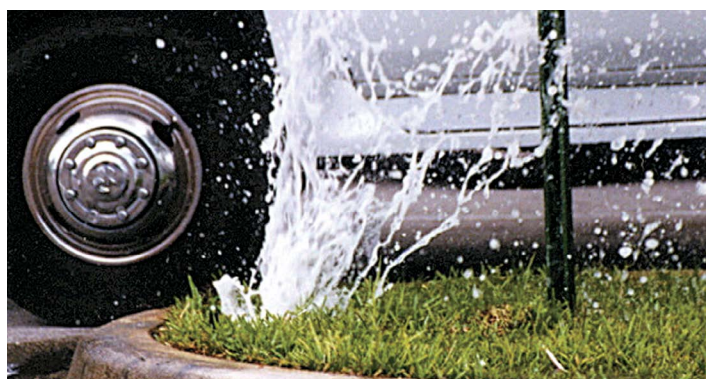
Figure 16. Water gushing from broken head.
