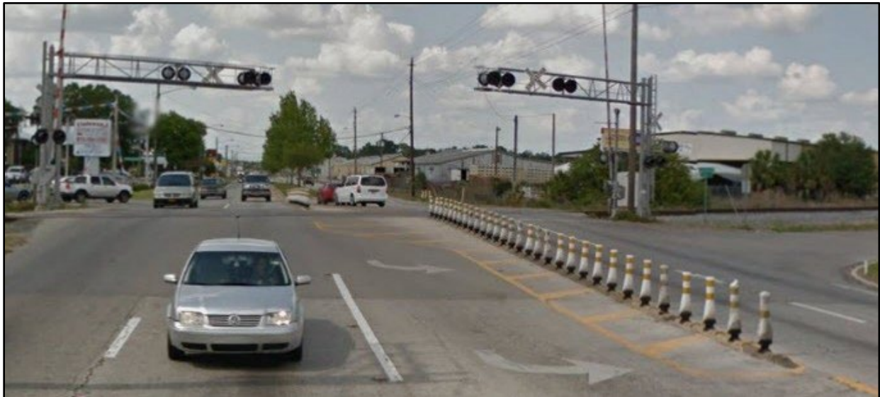
Alexander Street, SR 39A, Plant City, FL 1
