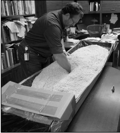
Figure 3-18. Spreading Bedding Material the.
