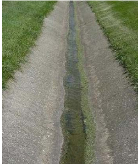
Paved or concrete channel
