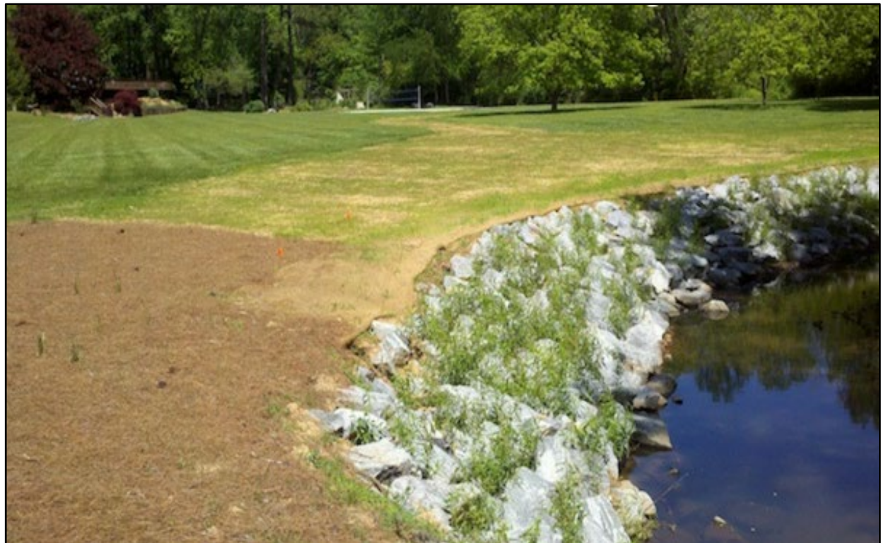
Figure 3.1 Rip Rap and Vegetation Hybrid Shoreline Example
