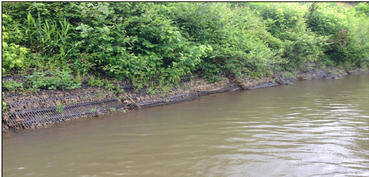
Figure 3.4 Example of Marine Mattress System (source: Tensar)
