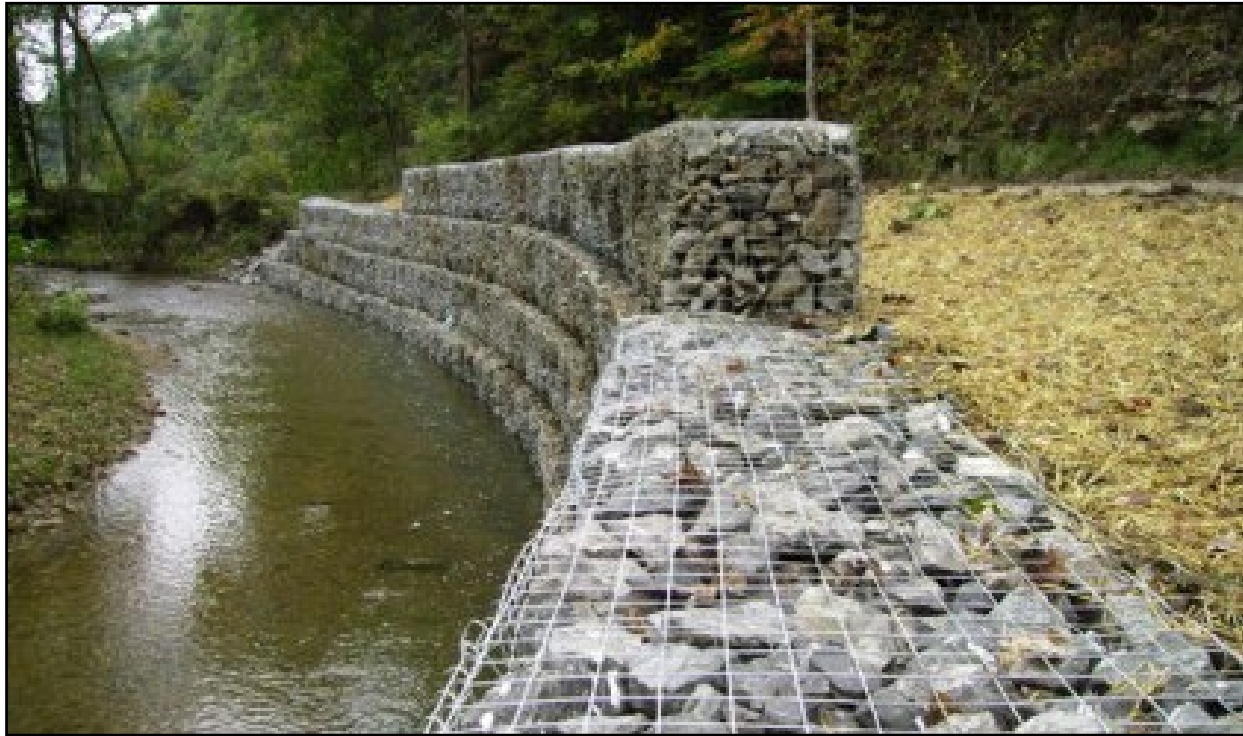
Figure 4.3 Example of Gabions
