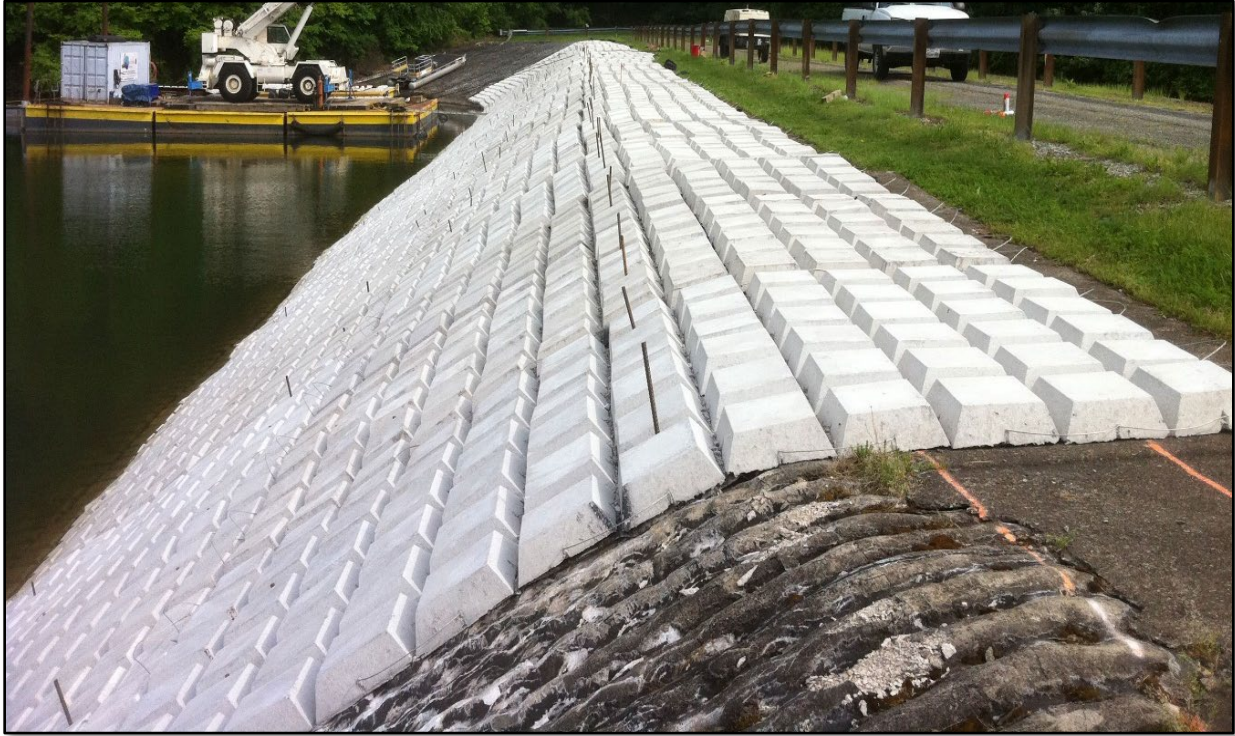
Figure 4.2 Example of Closed-Cell Articulated Concrete Blocks (source: Shoretec)
