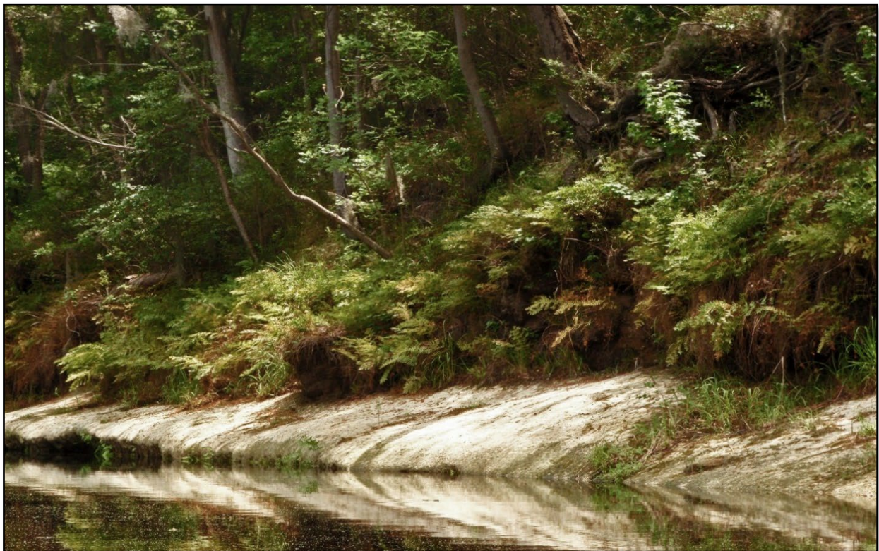
Figure 1.2 Example of Typical Shoreline Erosion Conditions (Gar Pond Tract)
