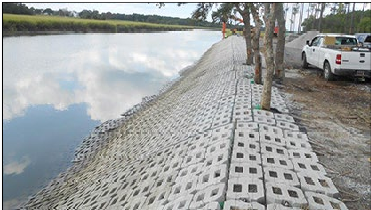
Figure 3.5 Example of Open-Celled Articulated Concrete Blocks (source: Shoretec)
