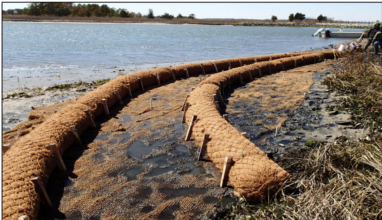
Figure 2.3 Example of Coir Logs Installation
