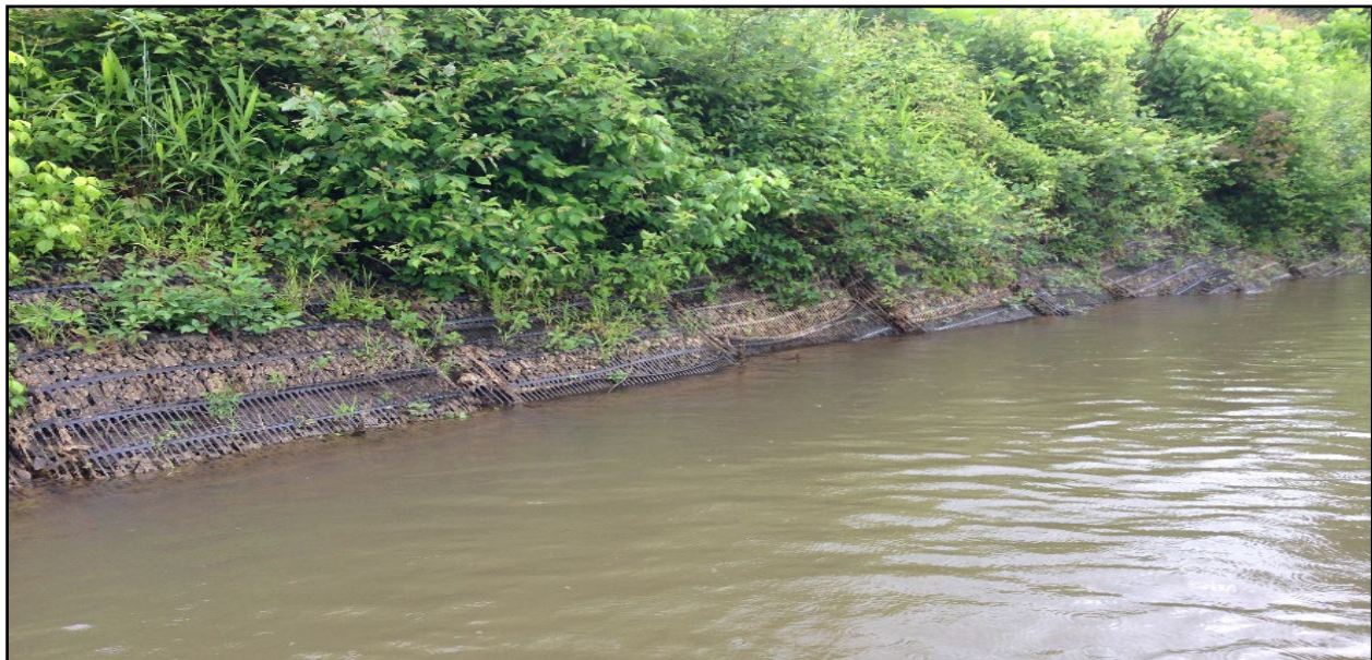
Figure 3.4 Example of Marine Mattress System (source: Tensar)
