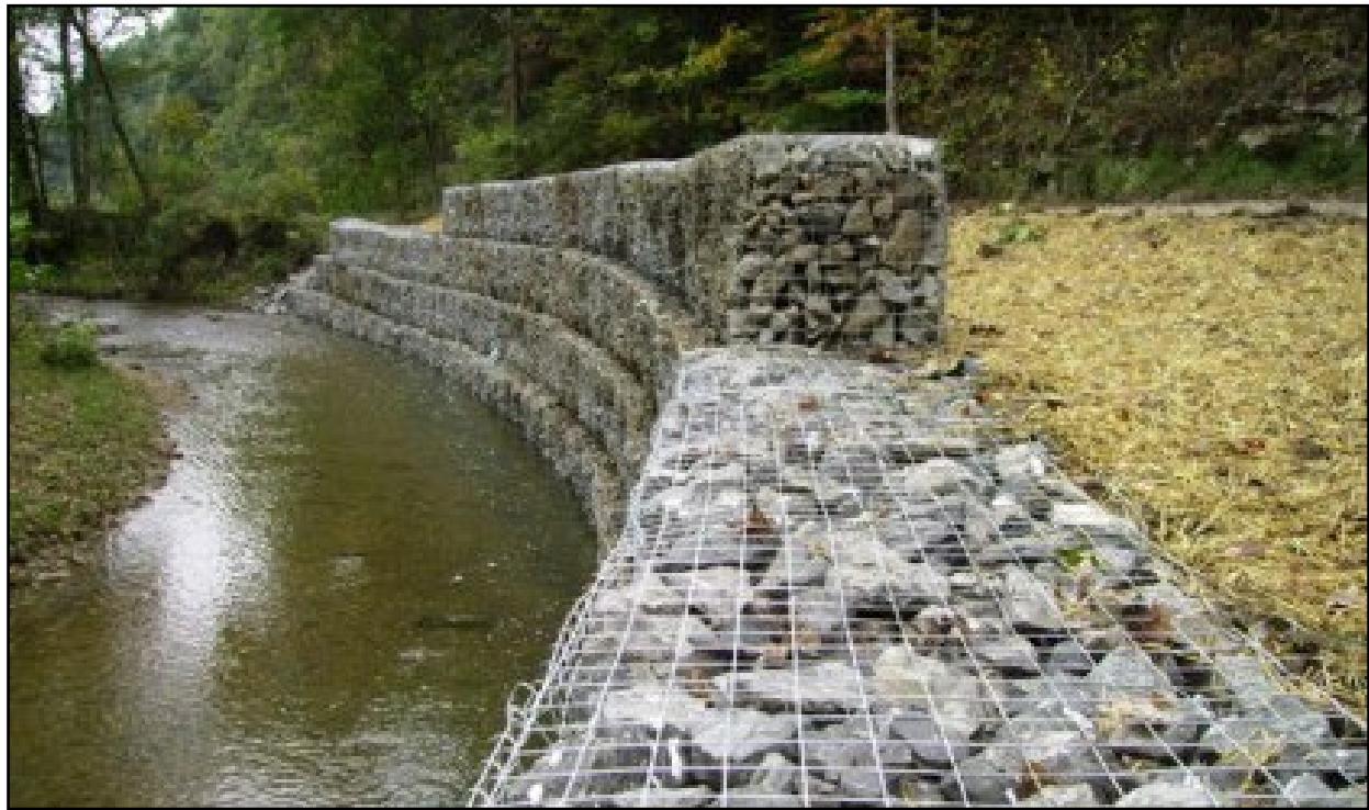
Figure 4.3 Example of Gabions
