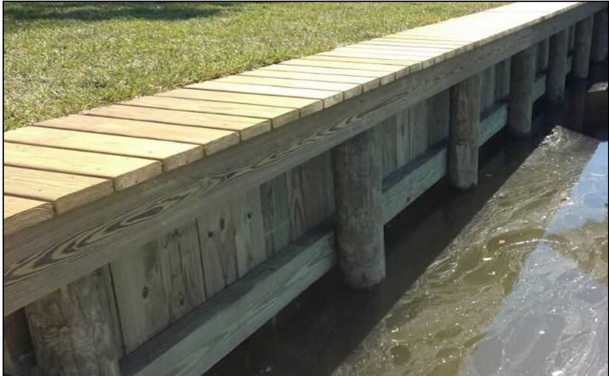
Figure 4.4 Example of Timber Bulkhead
