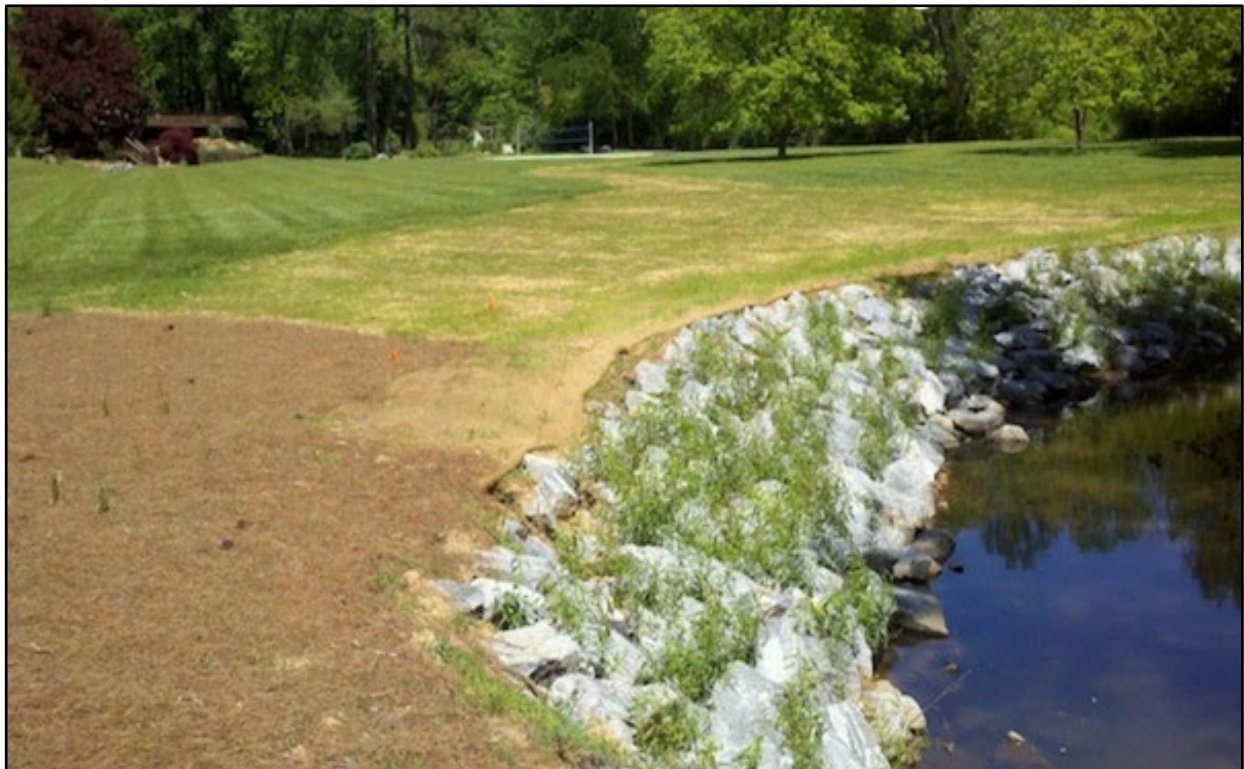
Figure 3.1 Rip Rap and Vegetation Hybrid Shoreline Example
